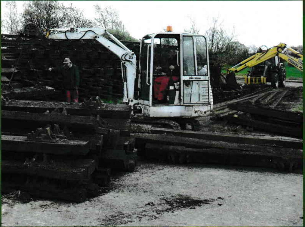
The Heavy gang removing the rails from the sleepers.
